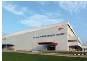
Proyek : Glico Owner : Wings Group Maincon : Jaya Obayashi
