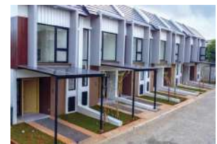
Proyek : Aksara Home Owner : PT. Syhthesis Development Maincon : PT. Maju Mapan Bangunindo
