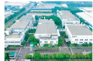
Proyek : Kansai Indonesia Owner : Kansai Paint Indonesia Maincon : Jaya Obayashi
