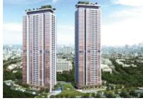
Proyek : The Pakubuwono Spring Owner : Pakubuwono Development Maincon : Total Bangun Persada, Tbk.
