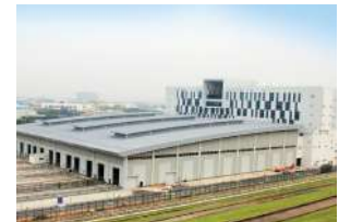
Proyek : LTA Depot Owner : Land Transport Authority Maincon : GS E&C Corp.
