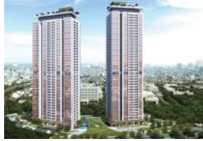
Proyek : The Pakuwono Spring Owner : Pakuwono Development Maincon : Total Bangun Persada, Tbk.
