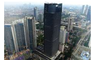
Proyek : Astra Tower Owner : PT Astra International Tbk. Maincon : Shimizu
