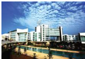
Proyek : UNIMAS, Sarawak Owner : University Malaysia Sarawak
