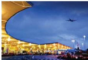
Proyek : Low Cost Carrier Terminal (LCCT) Owner : Government of Malaysia
