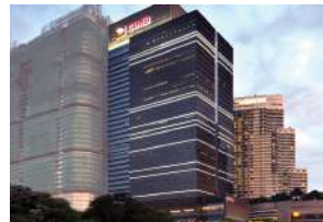
Proyek : CIMB 40 Story Office Block Owner : CIMB Maincon : MRCB Engineering
