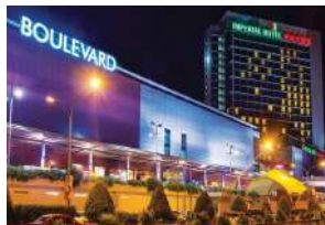
Proyek : Imperial Mall, Sarawak Owner : Imperial Group
