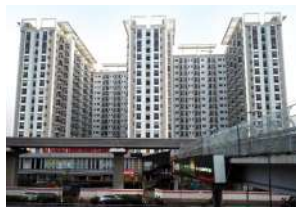
Proyek : Signature Park Grande Owner : PIKKO Group Maincon : PuLaintan BPK
