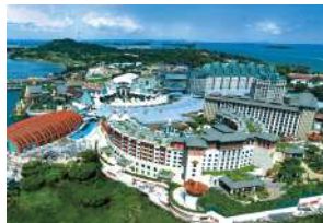
Proyek : Resort World Sentosa Owner : Genting Group Maincon : Sembawang Engineers
